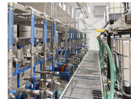
MEI's Turnkey Pump & Meter Stands automatically pull chemistry and/or micronutrients from mini-bulk tanks to add to the system blend.
