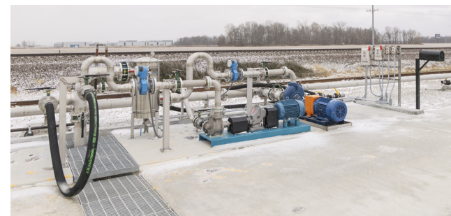
The new railcar unloading system allows Tipton to unload 5 railcars in 3 hours, which used to take a week via truck.
