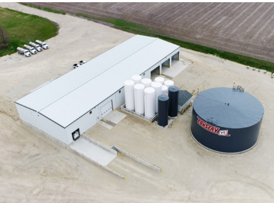
Conserv FS new liquid fertilizer facility can load five times the trucks, five times faster.
