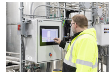
A conveniently located touchscreen panel allows employees to quickly create accurate batches.
