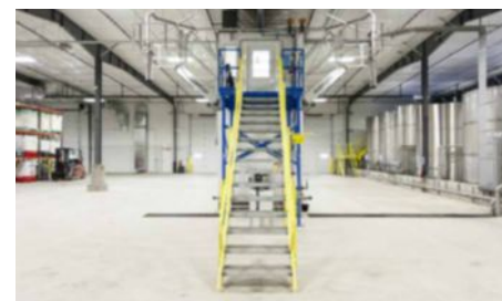
The new facility features 2 fully automated fertilizer & crop chemical bays that require only a single operator.
