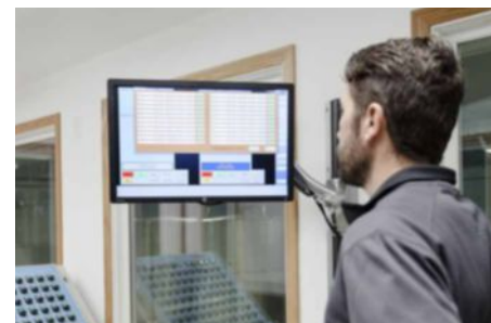
Inside the control room: MEI ICS 360 combined with Murray Interface offers a powerful, operator-friendly end-to-end automation solution.
