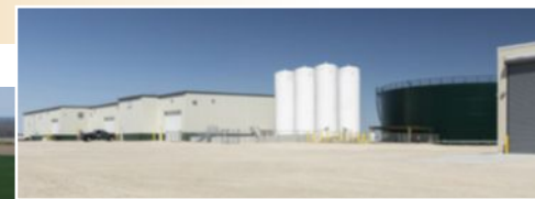
The new facility features both internal and external storage tanks with room for expansion.
