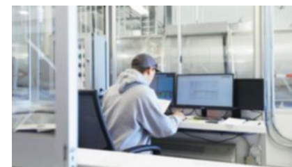
ICS ControlPro software manages the facility with an intuitive user-friendly interface. The same software manages the 24/7 unattended loadout bay for round-the-clock customer service.
