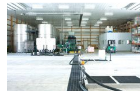
ABOVE: The floor plan was designed for efficiency, speed, as well as customer service. The large control room is air conditioned and employee-friendly.
