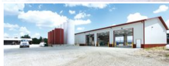
In addition to the indoor crop protection storage, the facility includes diked fertilizer tanks at the rear of the facility.
